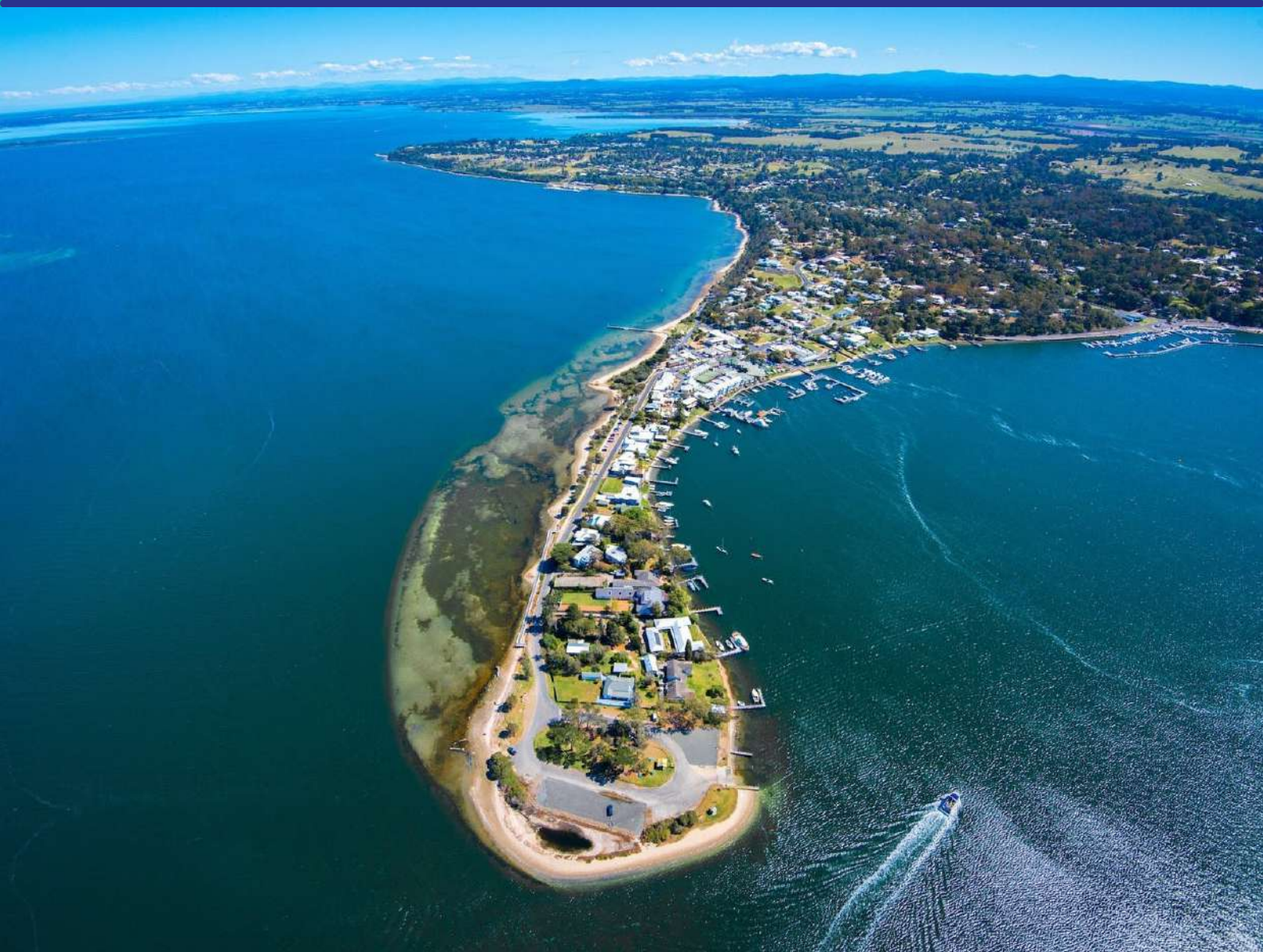
Lakes Entrance Victoria
